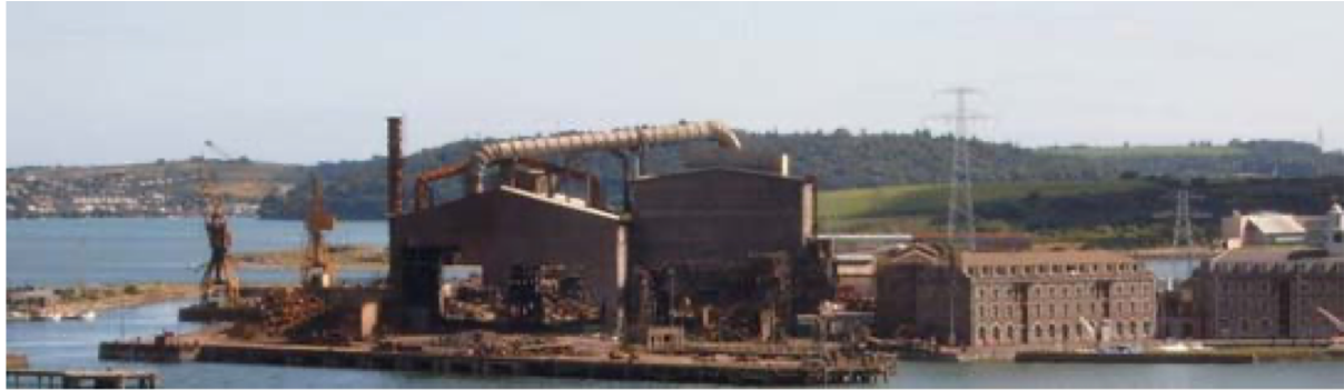
Irish Steel plant on Haulbowline Island Credit: Friends of the Irish Environment (2009) 9
